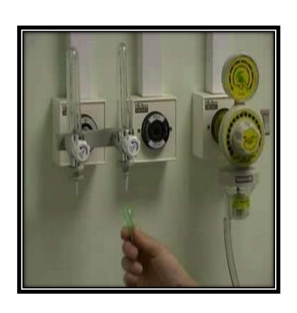
Medical gas outlets are always arranged in the same order from left to right and are identified by colour and the name of the gas.
